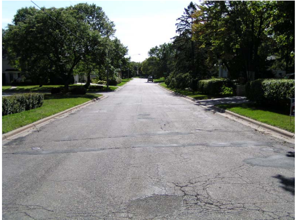
Photo 2. Existing Pavement Condition
