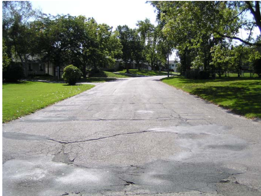
Photo 1. Existing Pavement Condition
